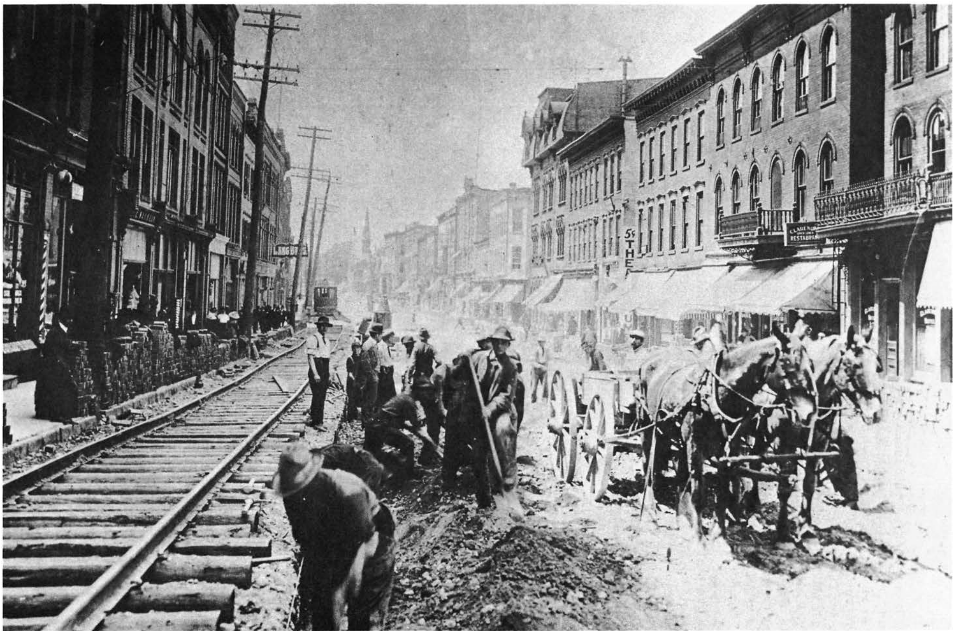
King Street, Berlin, c. 1910. Main business street of Berlin, from just north of the Queen Street intersection to the Water Street corner. The Berlin and Waterloo Street Railway Company was municipalized in 1908 and the line double-tracked in 1909-10. [Source: Kitchener Public Library]
