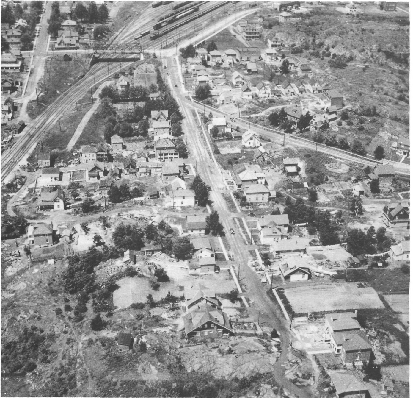
Sudbury, Portion of C.P.R. Yards, and adjacent housing, 1928. [NAPL, A169-66].
