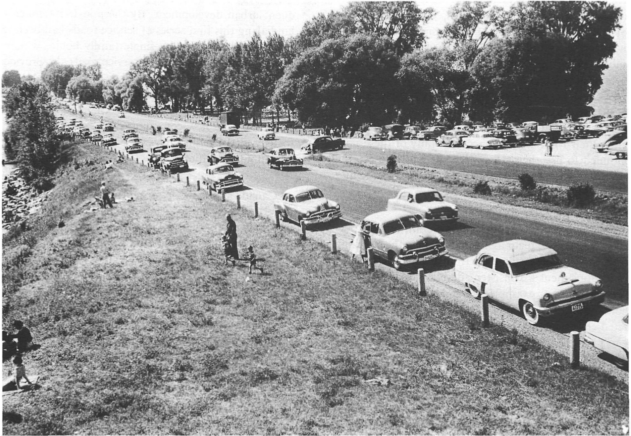
FIGURE 8. Picnicing along the Queen Elizabeth Way at Jordan Harbour; 1954.
