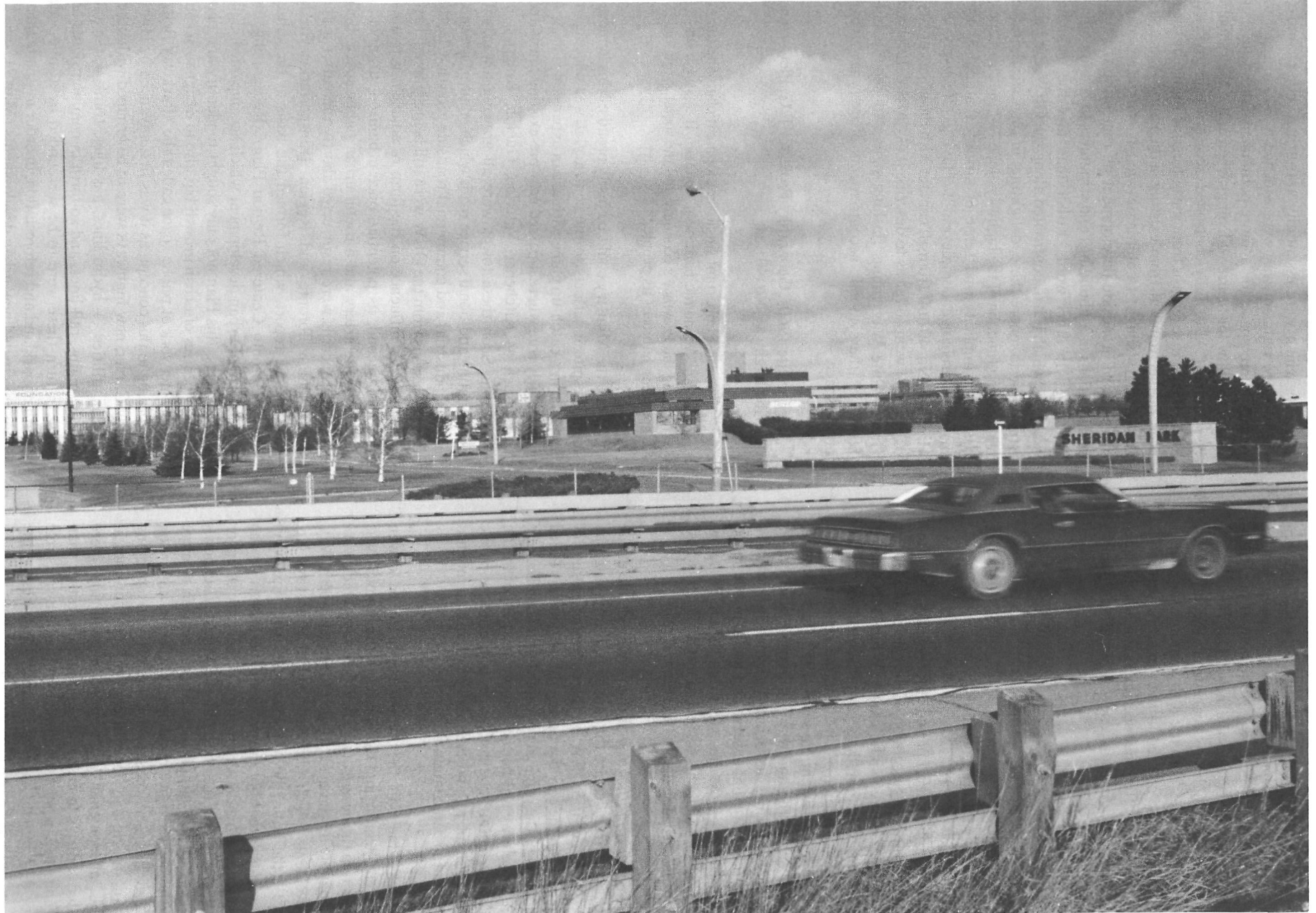
FIGURE 11. View of Sheridan Industrial Park, 1983, from the South Service Road, showing the entry gate and ceremonial drives.
