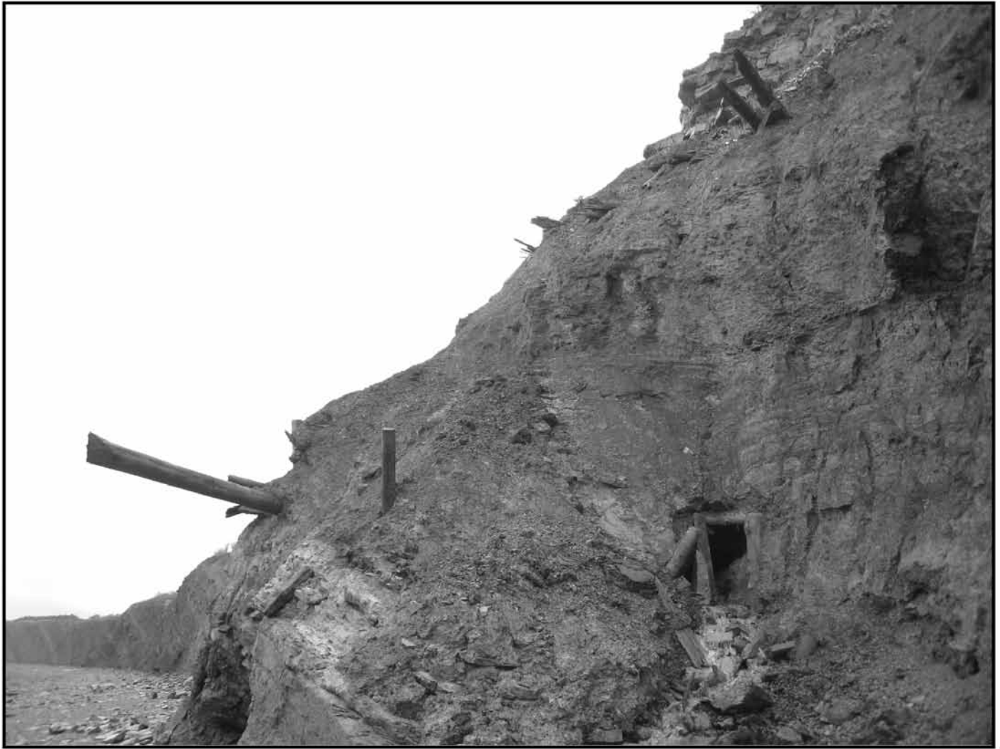
Fig. 4. The Fundy Seam at Joggins, showing timber pit props supporting a system of adits. These workings probably date from a later episode of mining in 1865, but according to Copeland (1958, p. 7) “old French workings” were visible at this site in the early nineteenth century (Jackson and Alger 1829).
