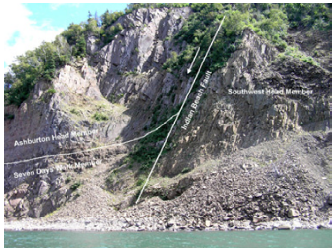
Fig. 5. A high-angle fault under the vegetation in this cliff face at Indian Beach separating lower Southwest Head Member (right side) from Seven Days Work (layered flows, lower left) and upper Ashburton Head (upper left) members of the Dark Harbour Basalt. The vertical offset is approximately 120 m based on positions of the basalt members. The steep joints are roughly parallel to the fault. The cliff face is about 80 m high, looking northeast.
