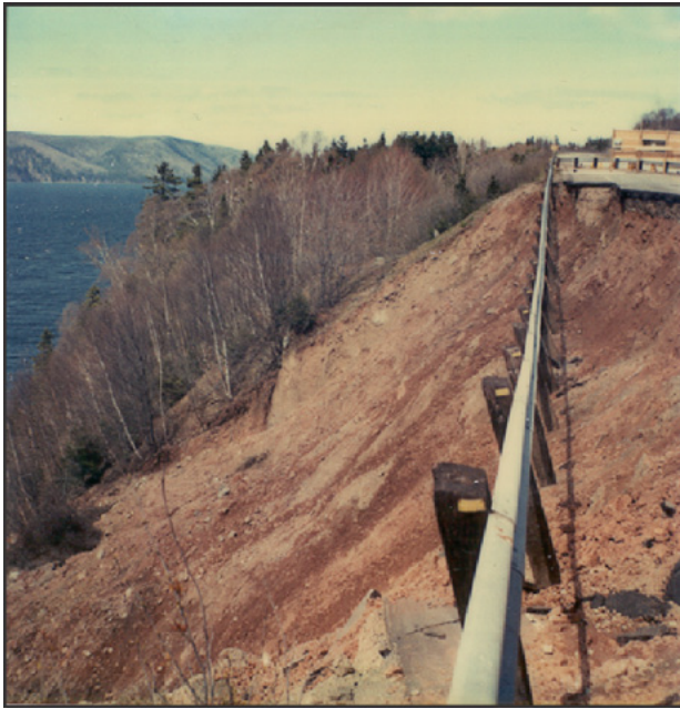
Figure 9. Debris-flow deposit at Kelly's Mountain, Cape Breton Island, Nova Scotia. This landslide has been characterized as a translational failure that developed into a debris flow.
