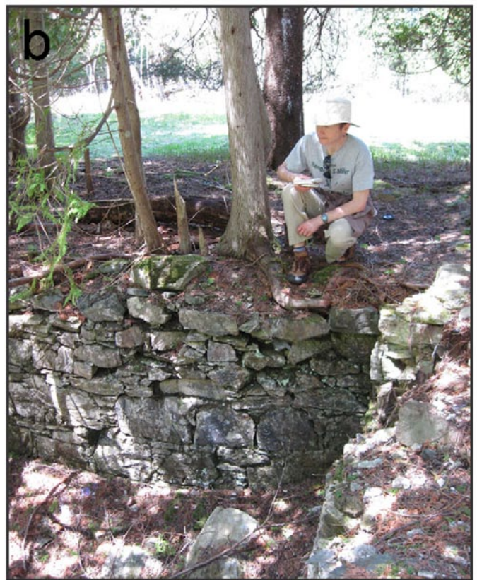
Figure 6. (a) The Joseph Armstrong house ca. 1890 (NBM 1961-25b); (b) Foundations of the Armstrong house in 2009 showing the 'ell', a part of the building with a cellar that lies perpendicular (behind) to the main house.
