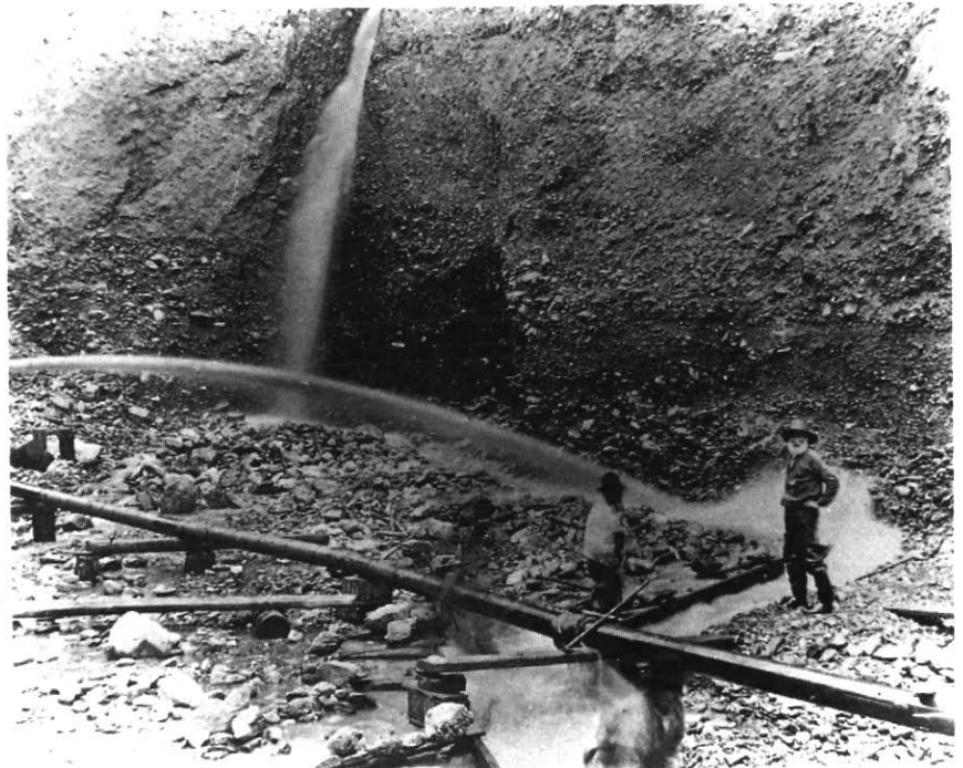
Figure 5 (a) (upper) Townsite at the base of Lowhee Creek just south of the present town of Wells, 1920s. (b) (lower) Hydraulic mining lodgement till and underlying gravels on the upper part of Lowhee Creek, 1930s.
