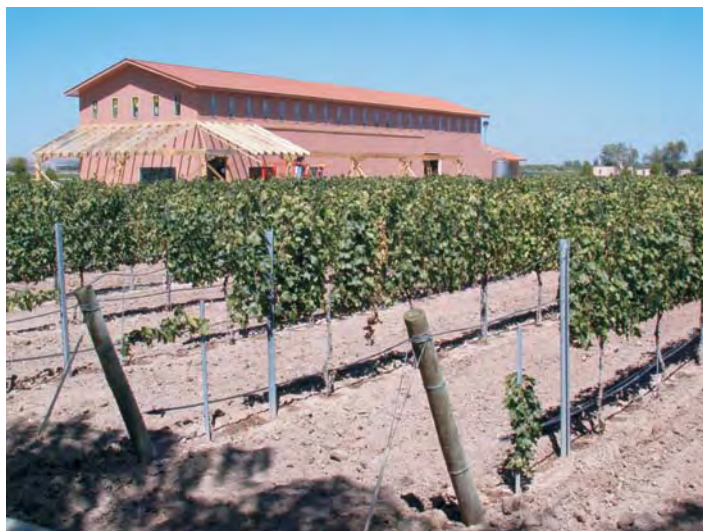
Figure 15. Zin Valle Vineyards with winery under construction in 2004; Mesilla Valley AVA.
