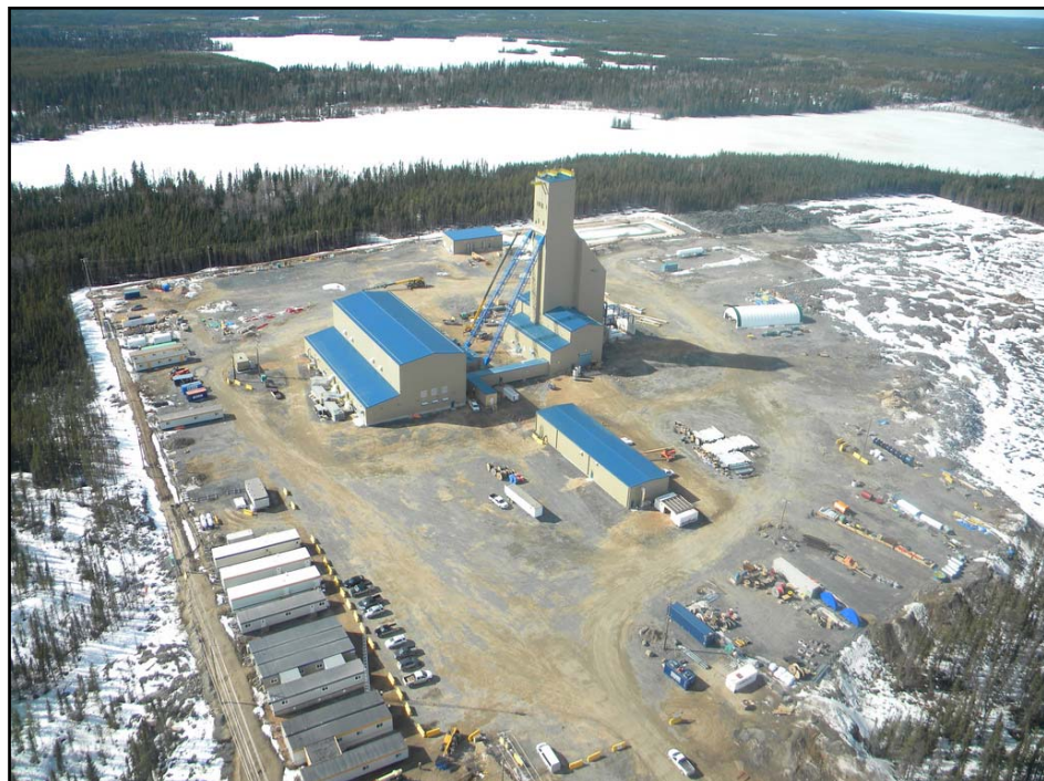
Figure 1. Aerial view of headframe and hoisthouse at Lalor Lake mine, November 2012.
