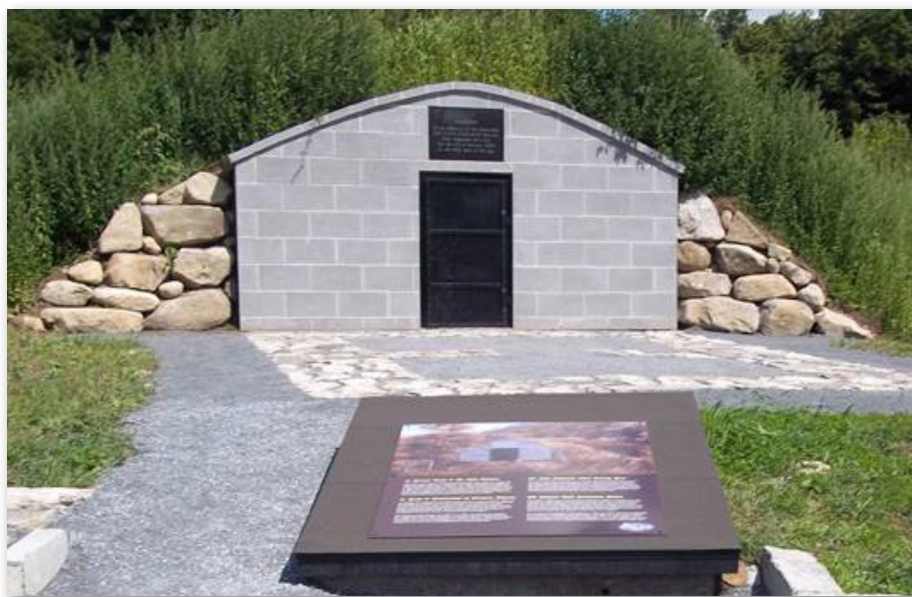
Restored Johnson Family Vault, mont Saint-Grégoire, 2014
