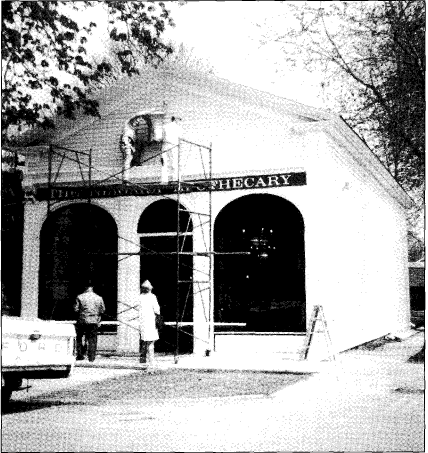
Constructing History: the mortar and pestle are affixed to the pediment, spring 1971. (OHF)
