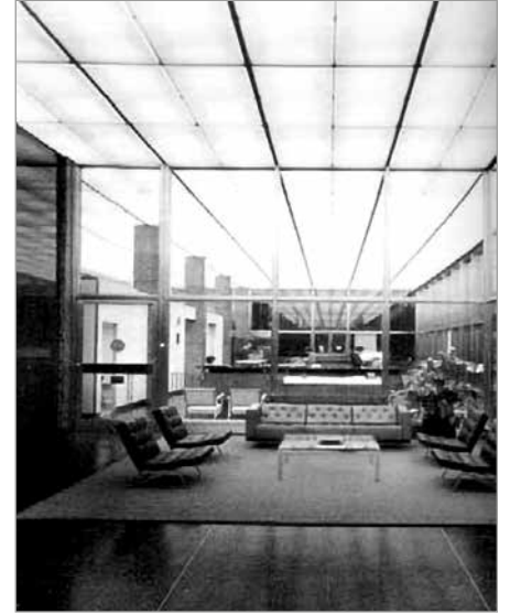
FIG. 7. MONARCH LIFE BUILDING 1961. | KESHAVJEE (ED.), WINNIPEG MODERN, P. 140.
