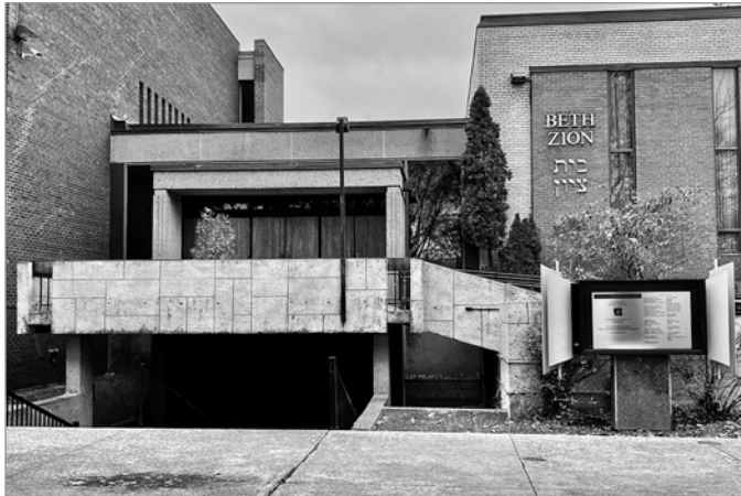
FIG. 15A. THE EXTERIOR OF BETH ZION SYNAGOGUE IN THE MONTRÉAL SUBURB OF CÔTE-SAINT-LUC, BUILT IN 1965 AND DESIGNED BY ANDRE VECSEI. | BARRY L. STIEFEL, NOVEMBER 2005.
