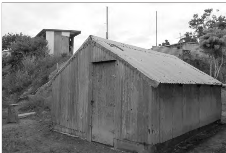
Fig. 2 Tormentera made of metal sheet in Adjuntas, Puerto Rico. Photograph by author.
