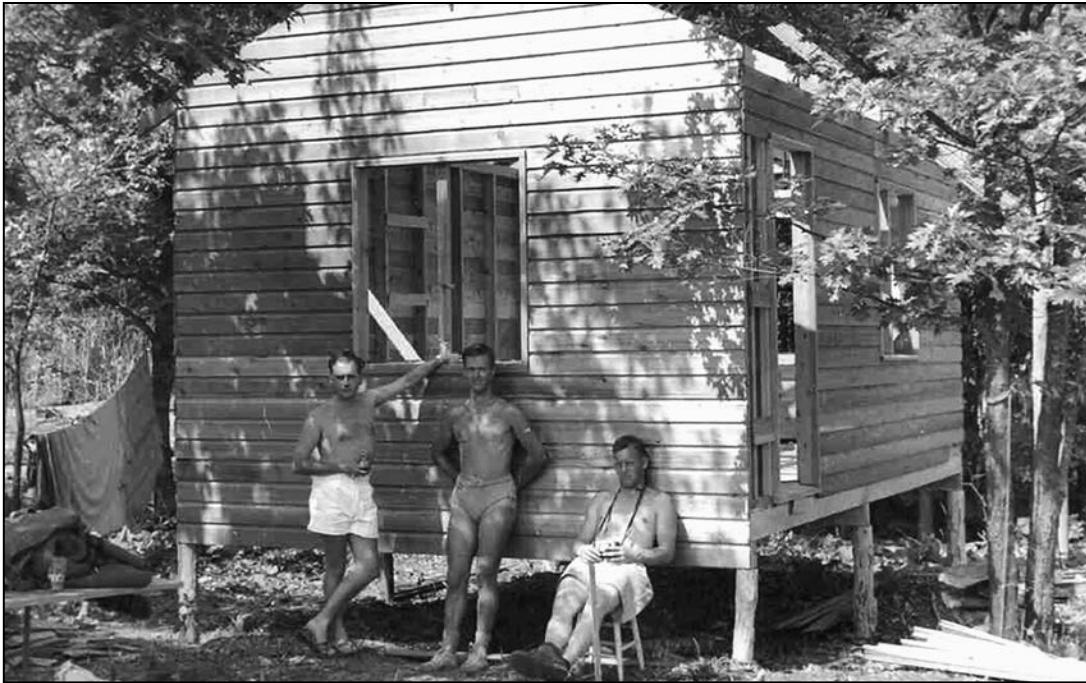
Three men take a break while building a simple cottage at Sixmile Lake, 1953. The postwar boom made cottage ownership possible for a wider portion of the general population. Photo courtesy of G. Crombie.
