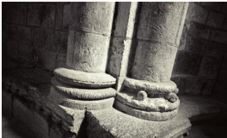
Photo 2: Columns in Nave
