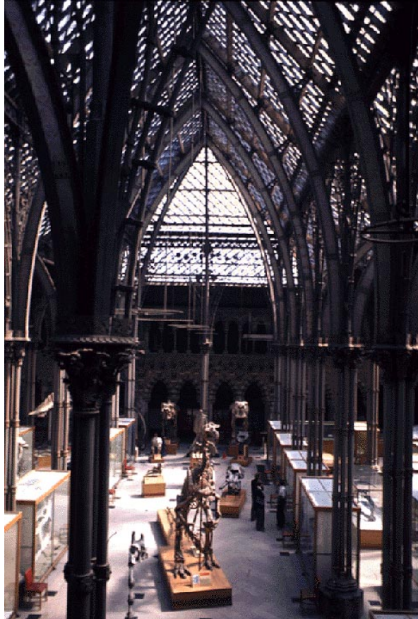
Figure 1: Oxford University Museum of Natural History, iron and glass roof, botanical capitals. Photograph by George Landow, 1977, courtesy of the Victorian Web at http://www.victorianweb.org/art/architecture/oxford/11.html
