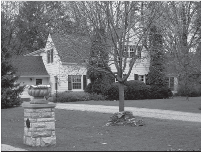
Figure 2: A typical Thorncrest Village home
